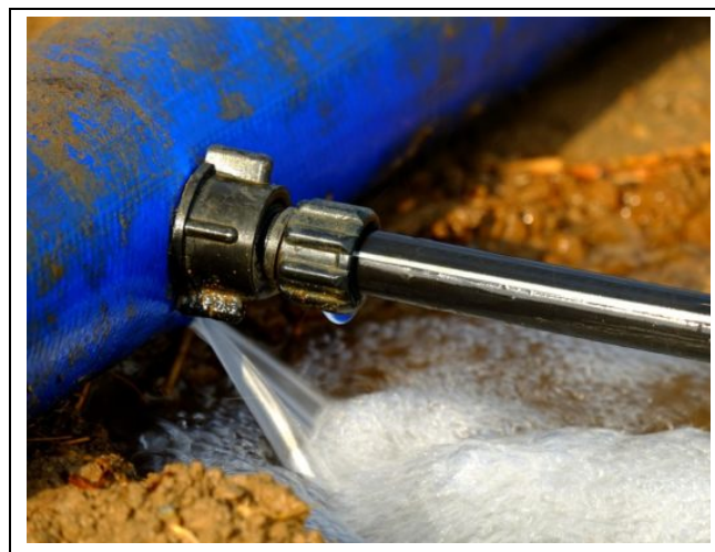
Figure 8: Illegal connection and leaking pipes
