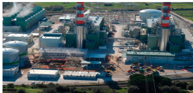
Figure 2: Maputo thermal power plant. The Maputo Thermal Power Plant (CTM) that operates according to two thermodynamic cycles (Gas and steam or Vapor) (EDM, u.d.)
