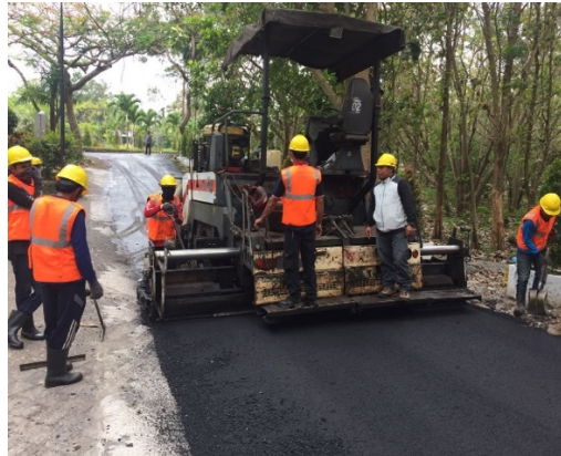
Figure 5: Plastic waste was tested as a mixture of asphalt for roads at the Udayana University campus, Jimbaran, Badung, Bali on Saturday (29/07/2017).
