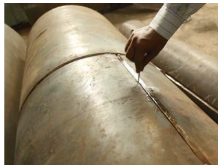
Figure 5: Root gap checking
