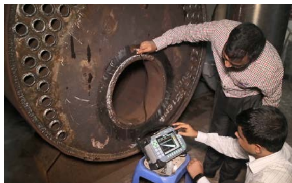
Figure 5: Ultrasonic test of welded joint
