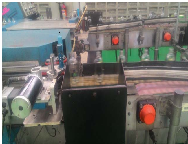
Figure 2: OLT reject chute
