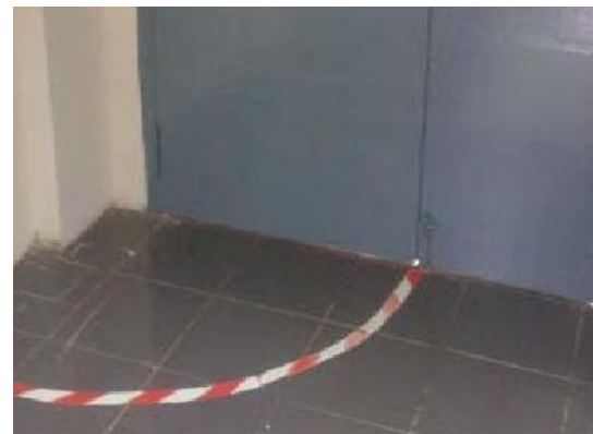
Figure.9 Safety sign indicating unsafe area
