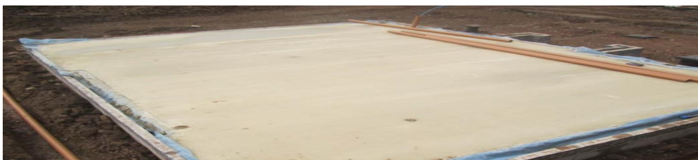
Figure 6. Concrete slab poured. DPM evident and lapping over internal block skin.
