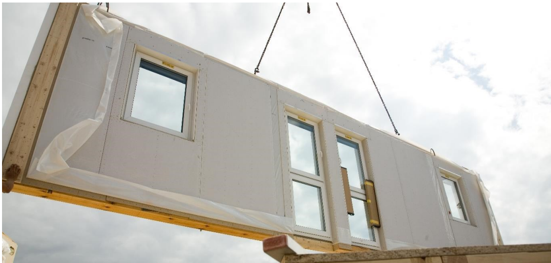
Figure 1: Part of the house built off – site and then transported to the site to assemble. (Brandt 2017)
