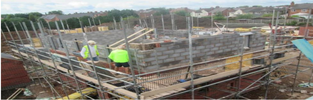
Figure 7. Brick and blockwork ongoing from ground to first floor level. Wall ties at reveals at each course and insulation appear satisfactory, maintain cavity cleanliness.
