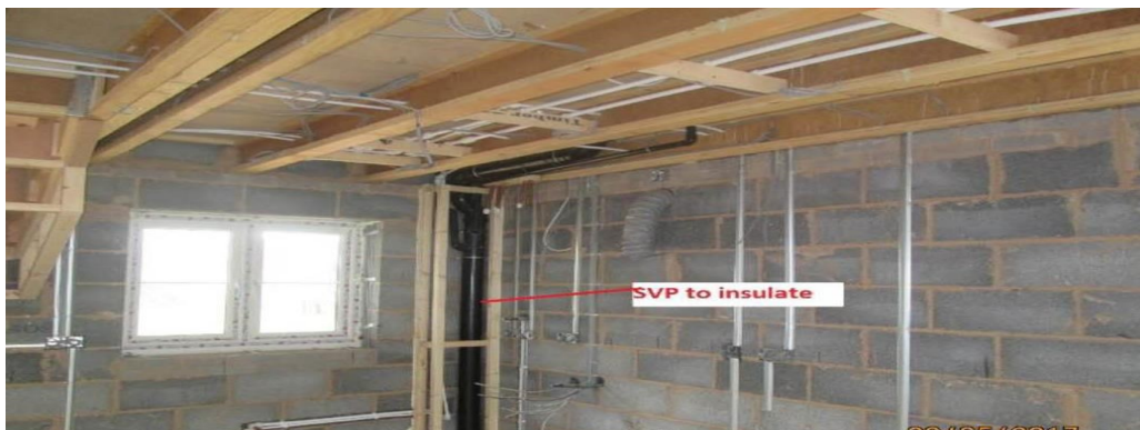
Figure 9. Insulation and wall plates straps are in place.
