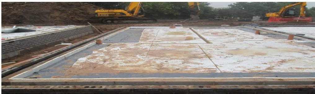
Figure 5. Engineering brick and block are in place, ready for the concrete block and beam to be placed on.
