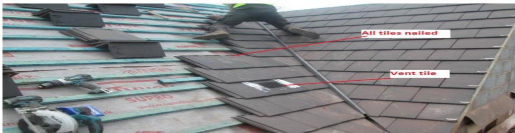
Figure 9. Roof tiling ongoing, noted all tiles being nailed, ridge vented, and VB lapped satisfactorily.
