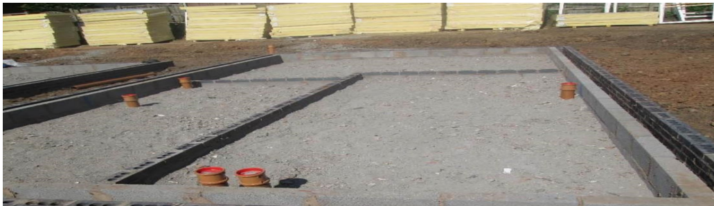
Figure 4. Cavities to fill before compaction of sub-base and sand blinding with membrane.
