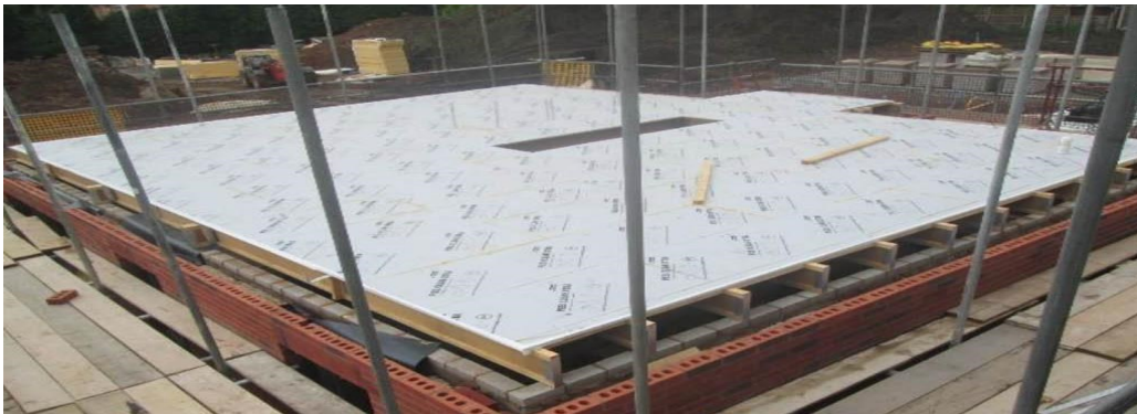
Figure 8. Joists and boarding fixed. Boards appear glued adequately. Joists bearing on walls adequately.
