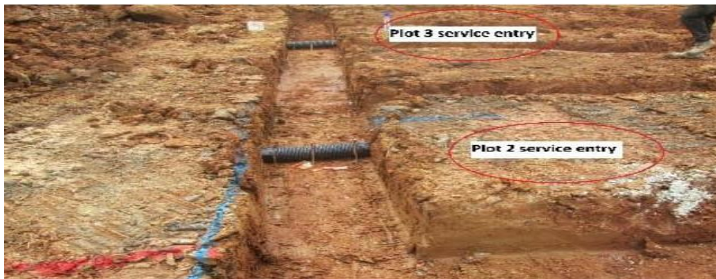
Figure 3. Foundations excavated to depth in clay, clean and dry ready for concreting. 150mm service entry ducts laid to front of property. Ducts pinned to prevent movement while concreting.
