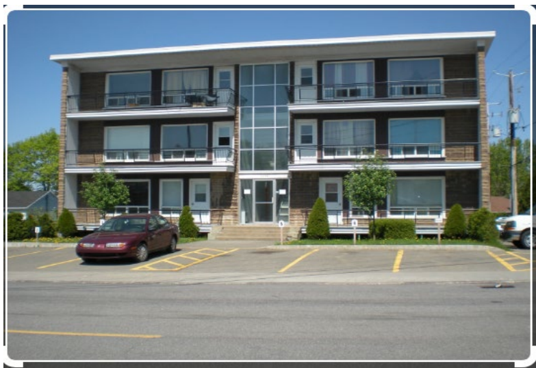
Figure 1. A Three-floor six-unit block of flats common in Zimbabwe ( http://www.pinintrest.com , 2023).
